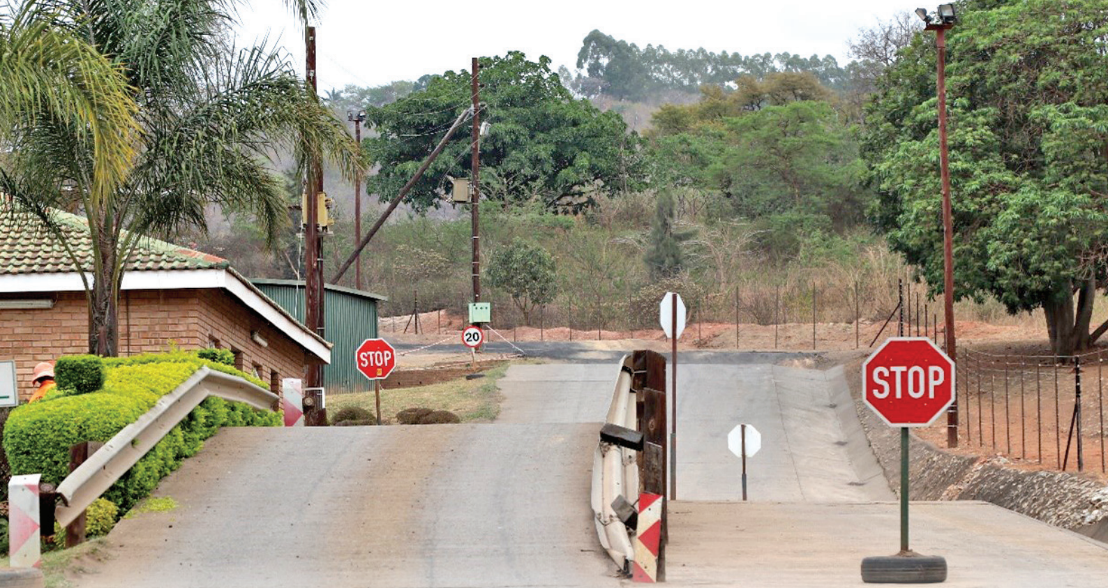
An impeccable landfill site in Tzaneen with an operative weighbridge, fence and complete infrastructure
